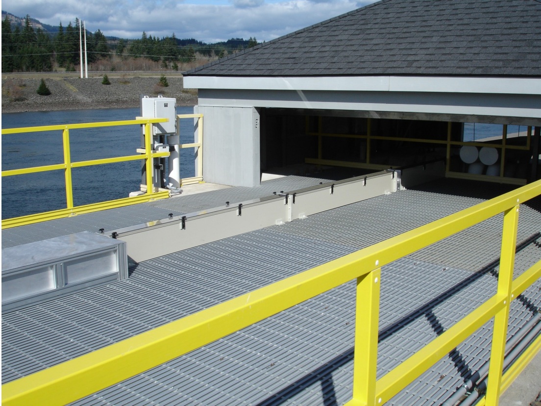
Figure 1. Upstream view of ARRT showing metal and plastic housing.
